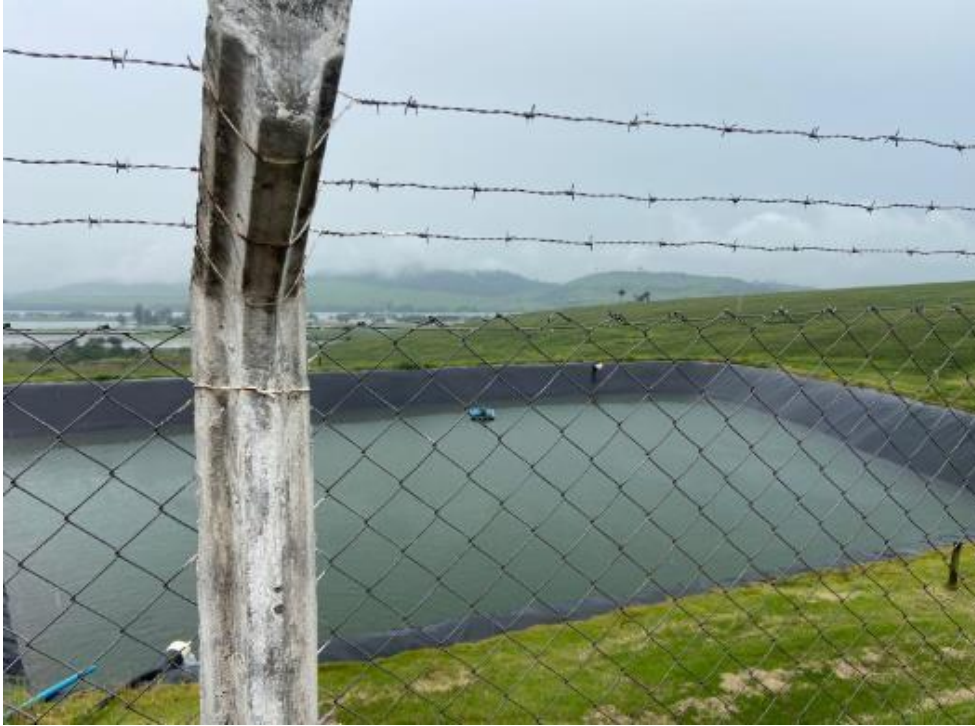
Figure 1. Rainwater catchment basin. (2023). Authors.
